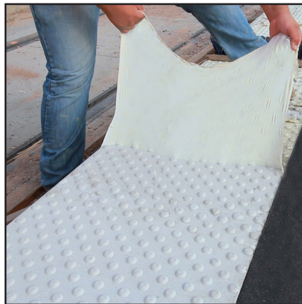
Removing Protective Covering (If applicable)
