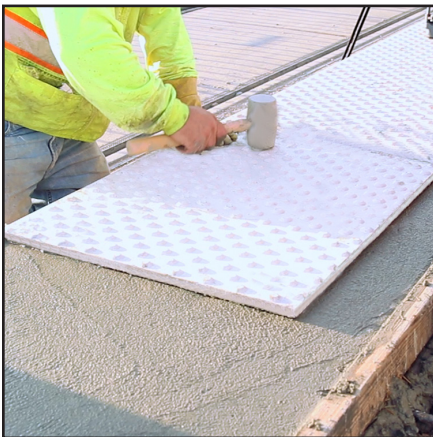
Step 4: Installing Dome-Tiles into Wet-Set (Fresh Concrete)
