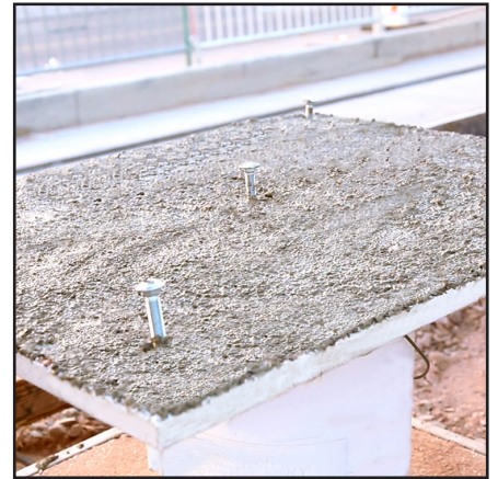
Step 3: Prepare Dome-Tiles for installation
