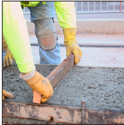
Step 2: Preparation of Wet Set (Fresh Concrete) for Dome-Tiles
